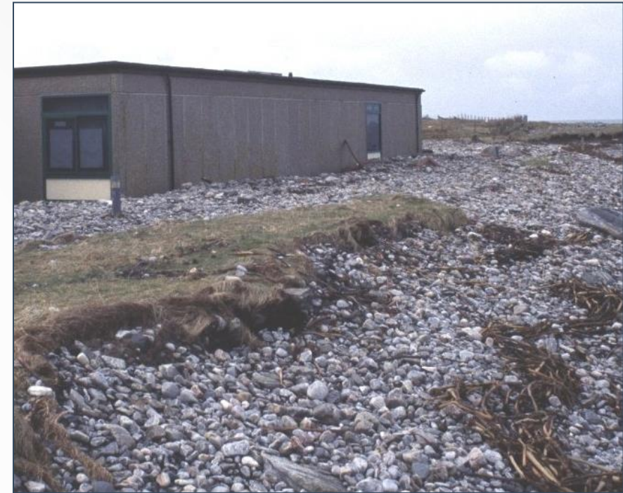
Old Balivanich School, Benbecula, Outer Hebrides, closed following storm damage >10m
